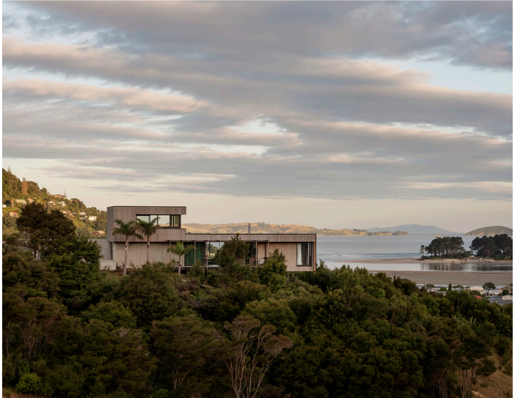
Stage 1 - The Cantilever House / Architect MDA Studio / Builder Turner Builders / Photographer Sam Hartnett
